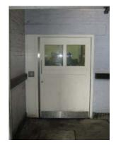
The final exit fire door at Bush Court has a missing bottom glazing panel; this must be replaced to maintain protection against fire and smoke entering the building from the Bin Store and Service Yard
