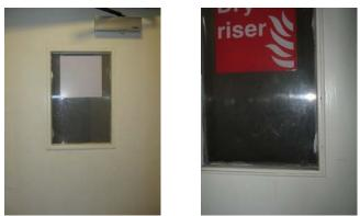
Most of the existing glazed panels are of Georgian wired glass held in by timber beads. There is no evidence of any intumescent sealing around the glass. Some glass panels have clearly been replaced, and in one instance the Georgian wired glass has been replaced by a thin sheet of clear plastic.
