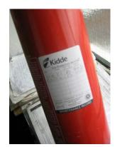
All three extinguishers show no evidence of having been checked within the last year; the dates of last checking shown on the extinguishers being  $19^{th}$  June 2000,  $2^{nd}$  November 2005 and  $6^{th}$  March 2007.
