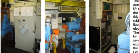
There is no fire detection within the lift motor rooms, but the rooms were both tidy and clean with rubber mats on the floor in front of electrical equipment. They were let down by the lack of serviced fire extinguishers and by the open cabinet to Lift A in Bush Court.
