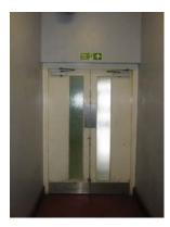
Between the bottom of the stairs and the lift lobby is a set of double opening doors. These are in serviceable condition but it is unlikely that they will provide fire or smoke protection to the escape route. They can be upgraded by the fitting of smoke seals but, as with the lobby/stair doors; no guarantee of performance can be given. These doors should, therefore, also be considered for replacement by a new doorset.
