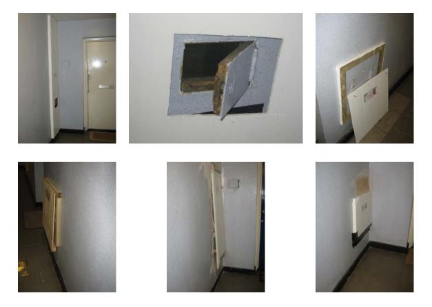
Some of the gas meter viewing windows have been broken and a small number had missing metal hatch covers. Where the glass was missing, many of the openings had been stuffed with paper to create a seal. All of the hatches have been overpainted and thus the hinges and, particularly, the locks function badly; there were also some missing locks.
